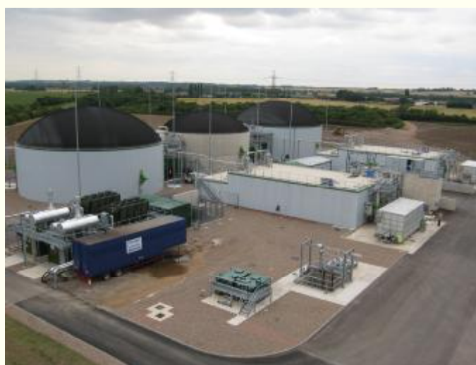
Biogas plant at Stoke Bardolph
